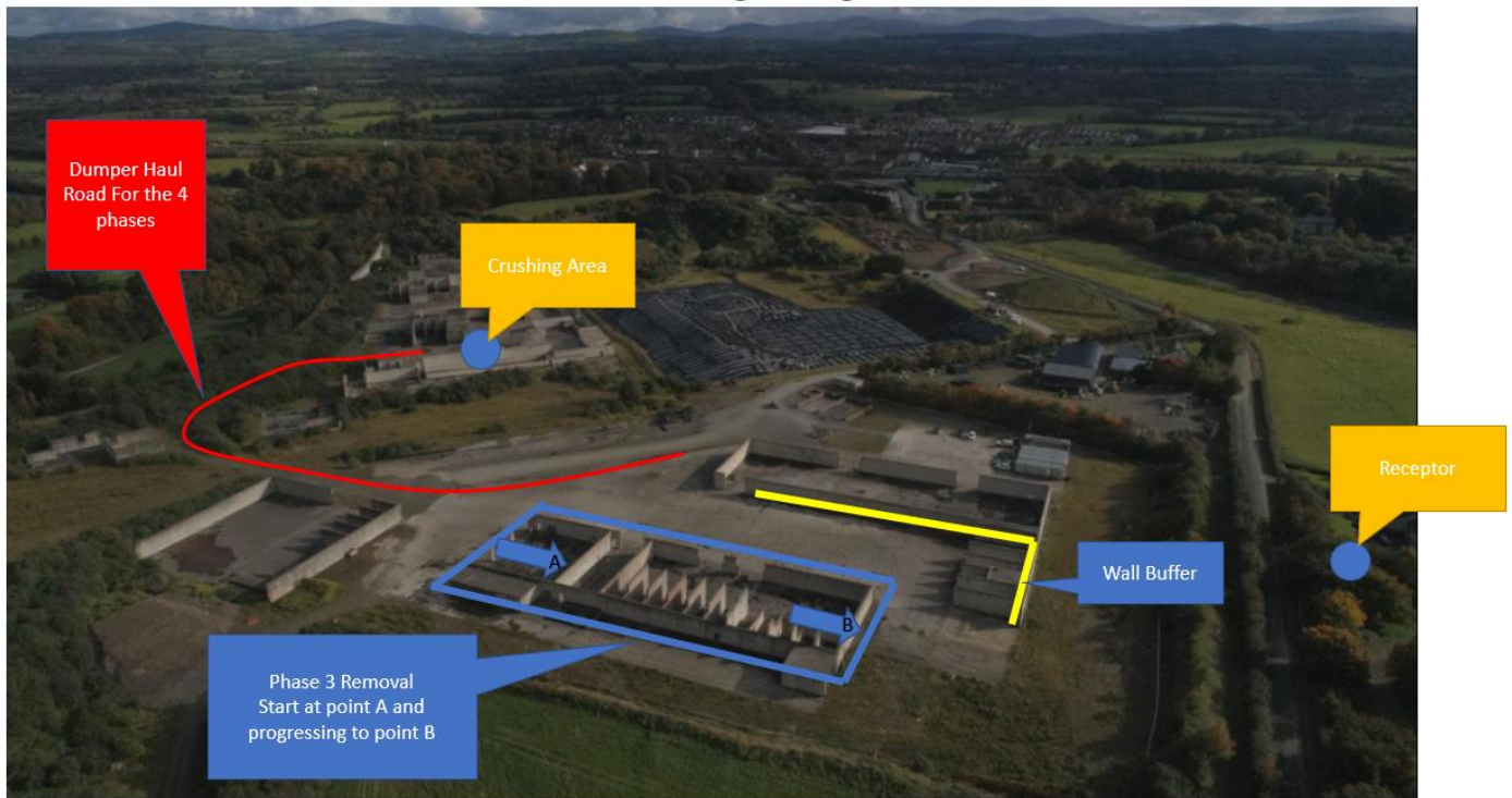
Figure 7-3 Phase 3 Zone 2A Demolition Works
