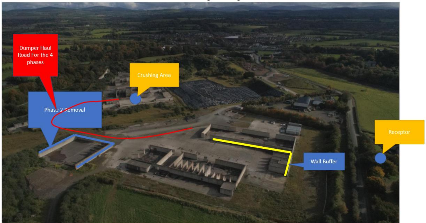
Figure 7-2 Phase 2 Zone 2A Demolition Works
