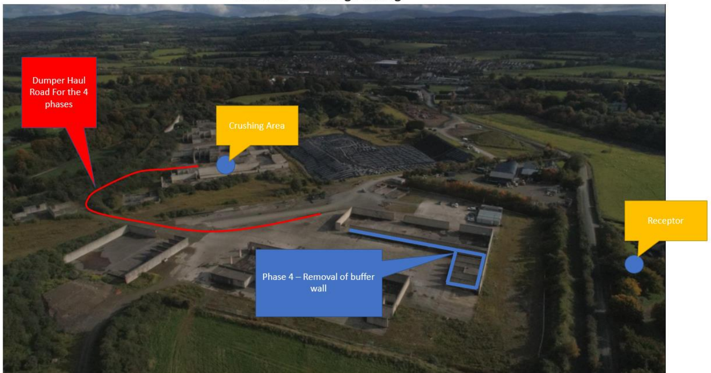
Figure 7-4 Phase 4 Zone 2A Demolition Works
