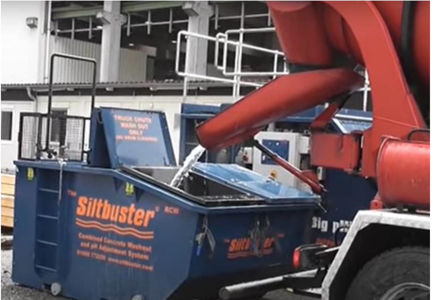
Figure 5-2 Siltbuster in operation
